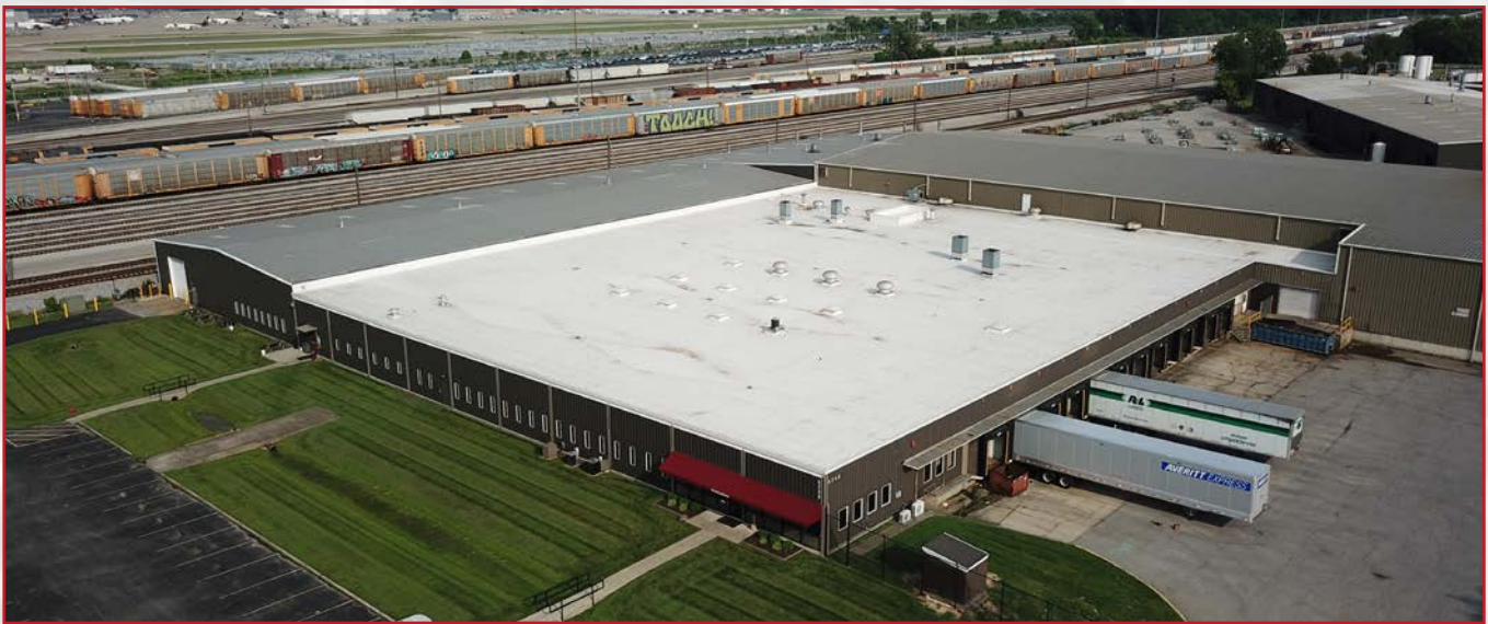
Aerial view of the WireCrafters facility.
