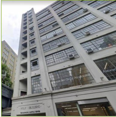
508-516 & 518-534 West 26 th Street, New York, NY NYSERDA Funding for LL97 Study Annual Savings: $428,944 GHG Reductions: 770.8 Tons of Co2 Project Area: 146,416 Square Feet
