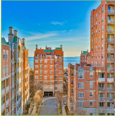
Oceana Condo, Brooklyn, NY (15 Bldgs) LL87, Energy Audit & RCx Annual Savings: $434,291 Project Area: 1,178,291 Square Feet
