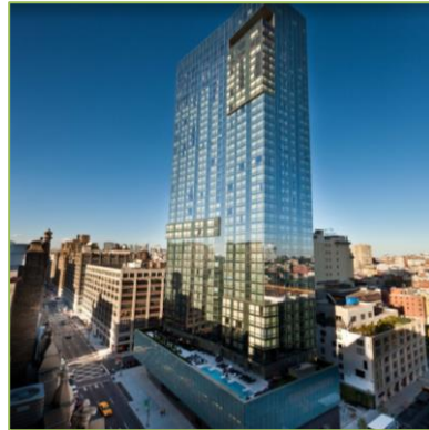
The Dominick Hotel, New York, NY LL87, Energy Audit & RCx Annual Savings: $451,185 Project Area: 386,078 Square Feet
