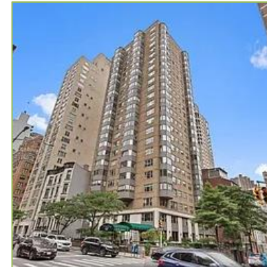
The Carlton Regency, New York, NY 100% NYSERDA Funding for LL87, LL97, MEP Design Annual Savings: $199,564 GHG Reduction: 500 Ton CO 2 Project Area: 242,383 Square Feet
