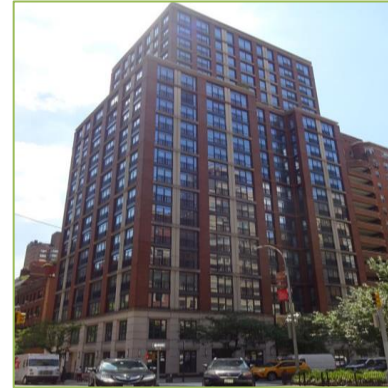
45 Park Avenue, New York, NY 100% NYSERDA Funding for LL97 & LL87 Study Annual Savings: $126,568 GHG Reduction: 143.30 Ton CO 2 Project Area: 118,614 Square Feet
