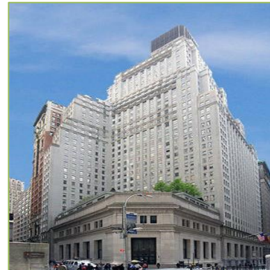
15 Broad Street, New York, NY Annual Savings: $519,058 Project Area: 810,798 Square Feet
