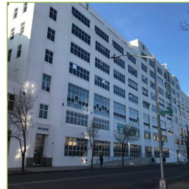
Pfizer Building, Brooklyn, NY LL87, Energy Audit & RCx Annual Savings: $1,149,714 Project Area: 574,055 Square Feet
