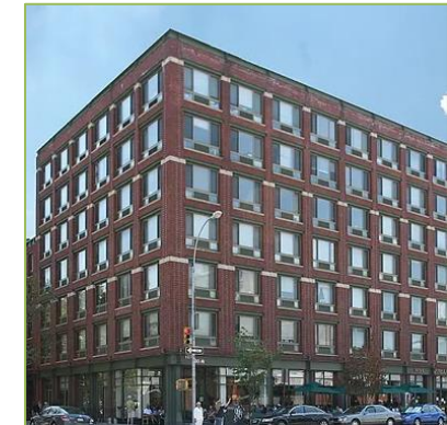
460 West 20 th Street, New York, NY 100% NYSERDA Funding for LL97 Study Annual Savings: $89,105 GHG Reduction: 134.38 Ton CO 2 Project Area: 68,260 Square Feet
