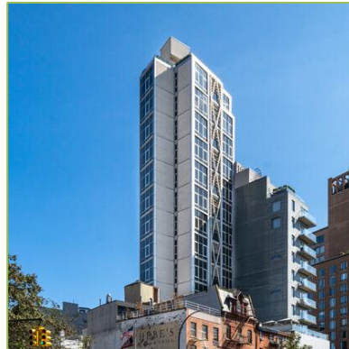
52 E 4 th Street, New York, NY NYSERDA Funding for LL97 Study Annual Savings: $50,742 GHG Reduction: 62.02 Ton CO 2 Project Area: 26,790 Square Feet
